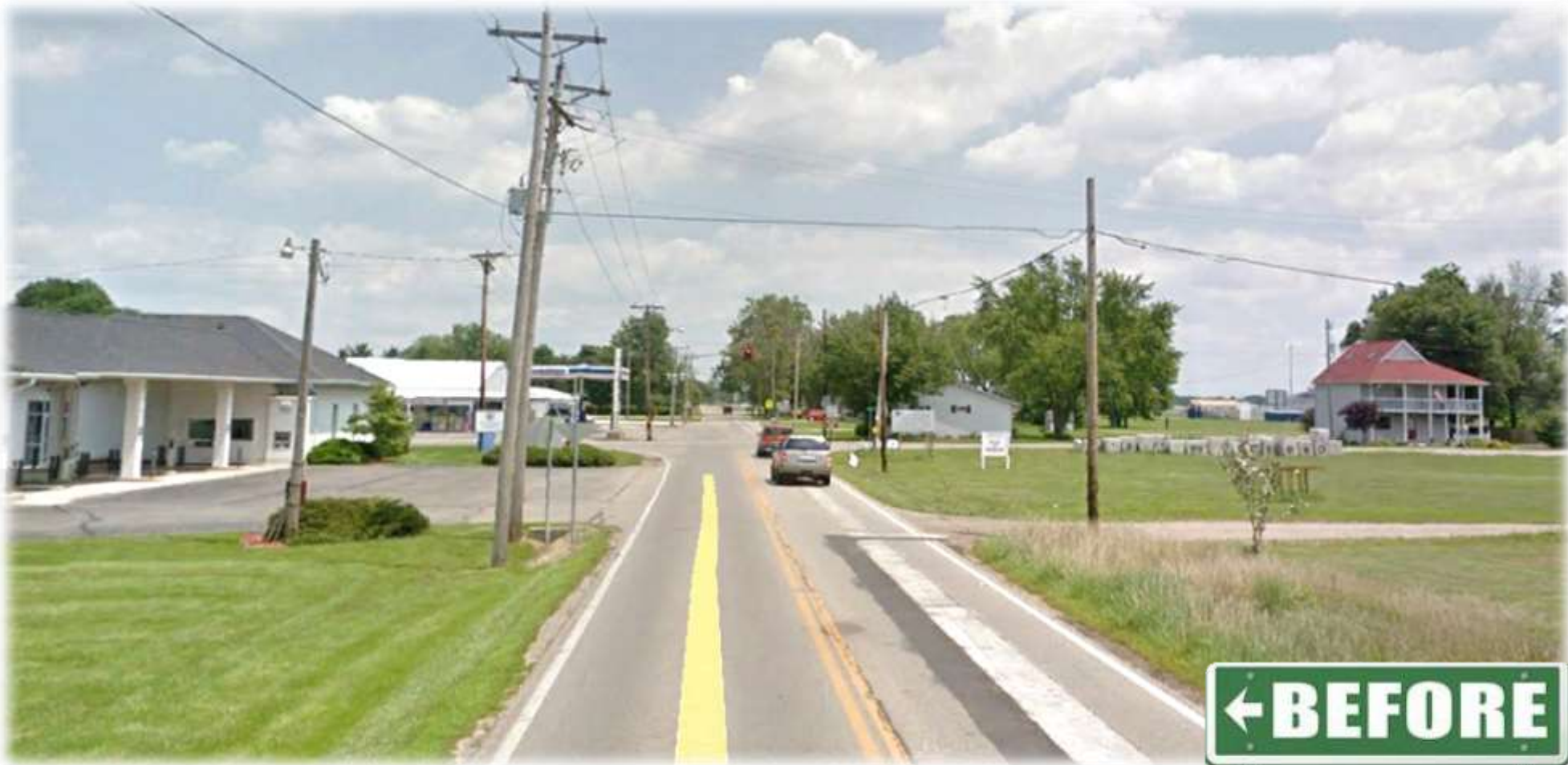
Photos from 2014 – State Route 752 west of Long Street
