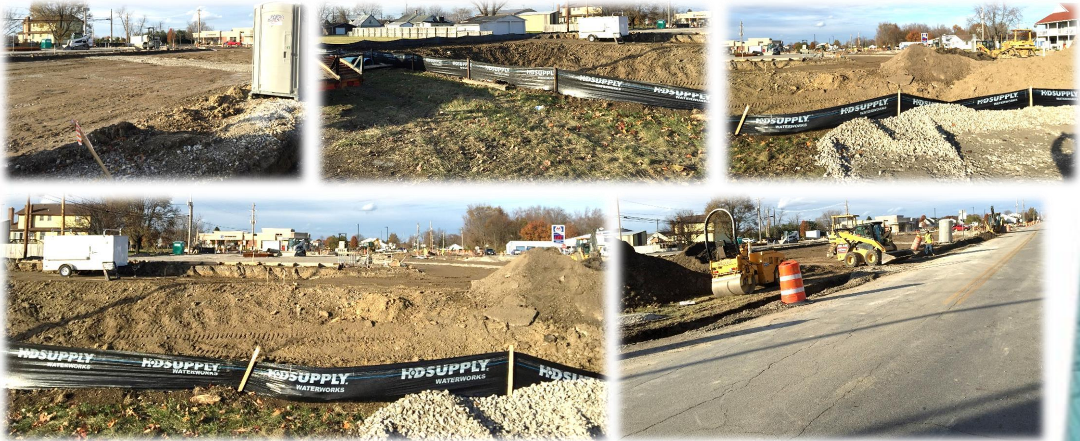
Photos from November 29, 2016 East to West South of 752 Corner Lot
