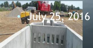
Transferring water from the Post Air/UV tank to the West half of the Aerobic Digester in preparation for leak testing.
