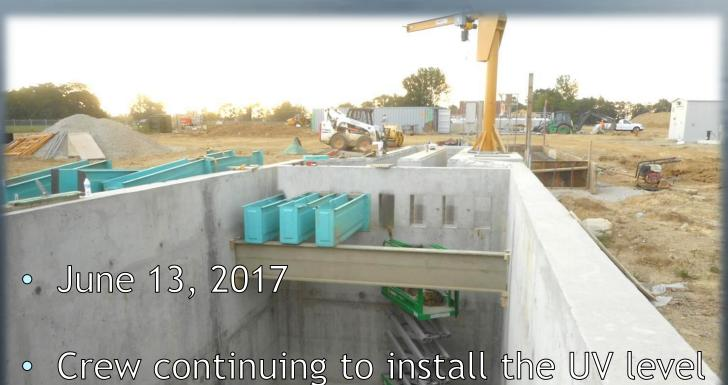
Crew continuing to install the UV level control weirs in the Post Air/UV tank.
