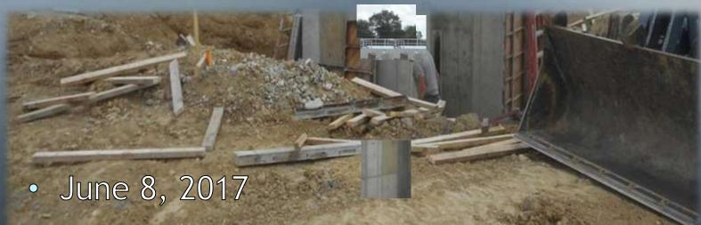
Crew stripping the concrete forms form the walls of the Clarifier Splitter Box.
