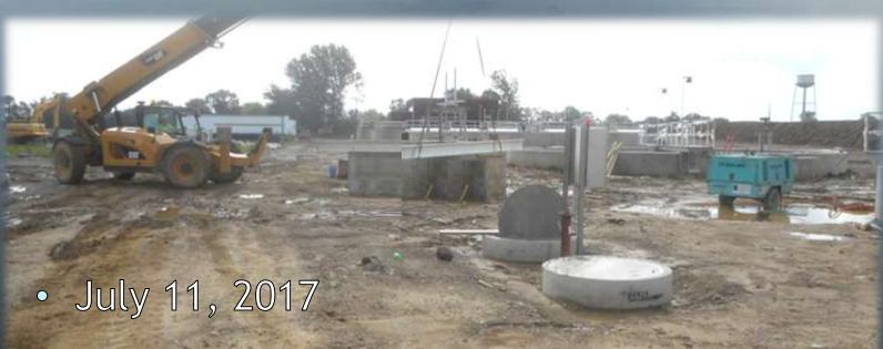
Crew installing one of the Aluminum I-Beams for the grating platform on the Clarifier Splitter Box.
