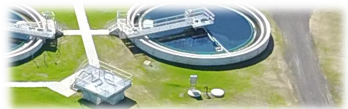
Scum Pump Station and Valve Vault
