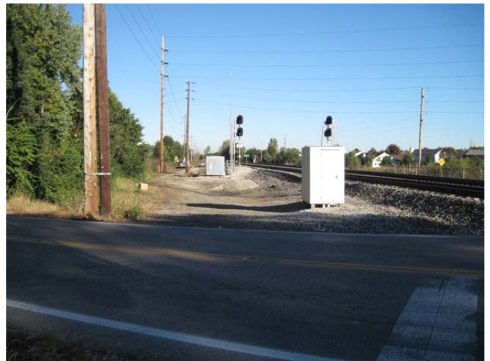
Photo 12: Norfolk & Southern RR right-of-way, across Ohio 752. Viewing north.
