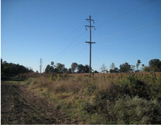
Photo 9: Electrical power lines running along Site eastern boundary. Viewing SSW.
